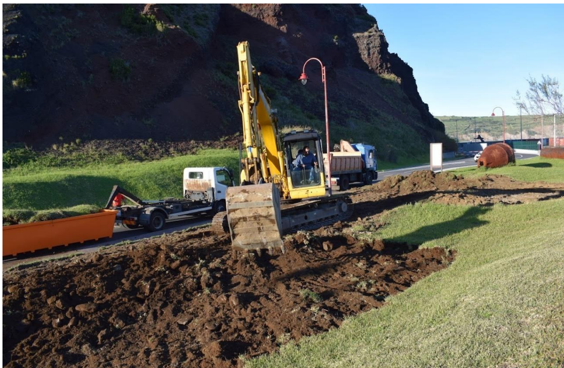
Figure 1 - Heavy Machinery works in Monte da Guia Intervention Area
